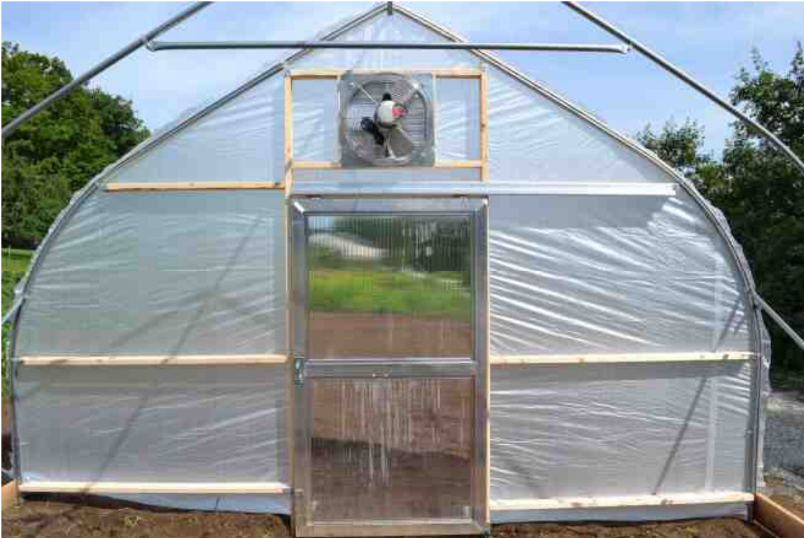
This is the exhaust fan
