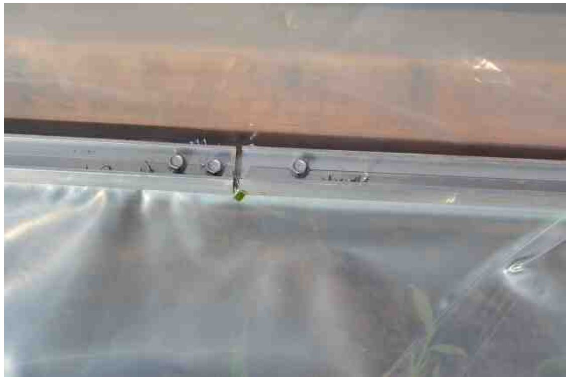
The two screws are where the tubes connect with the swedged connection
