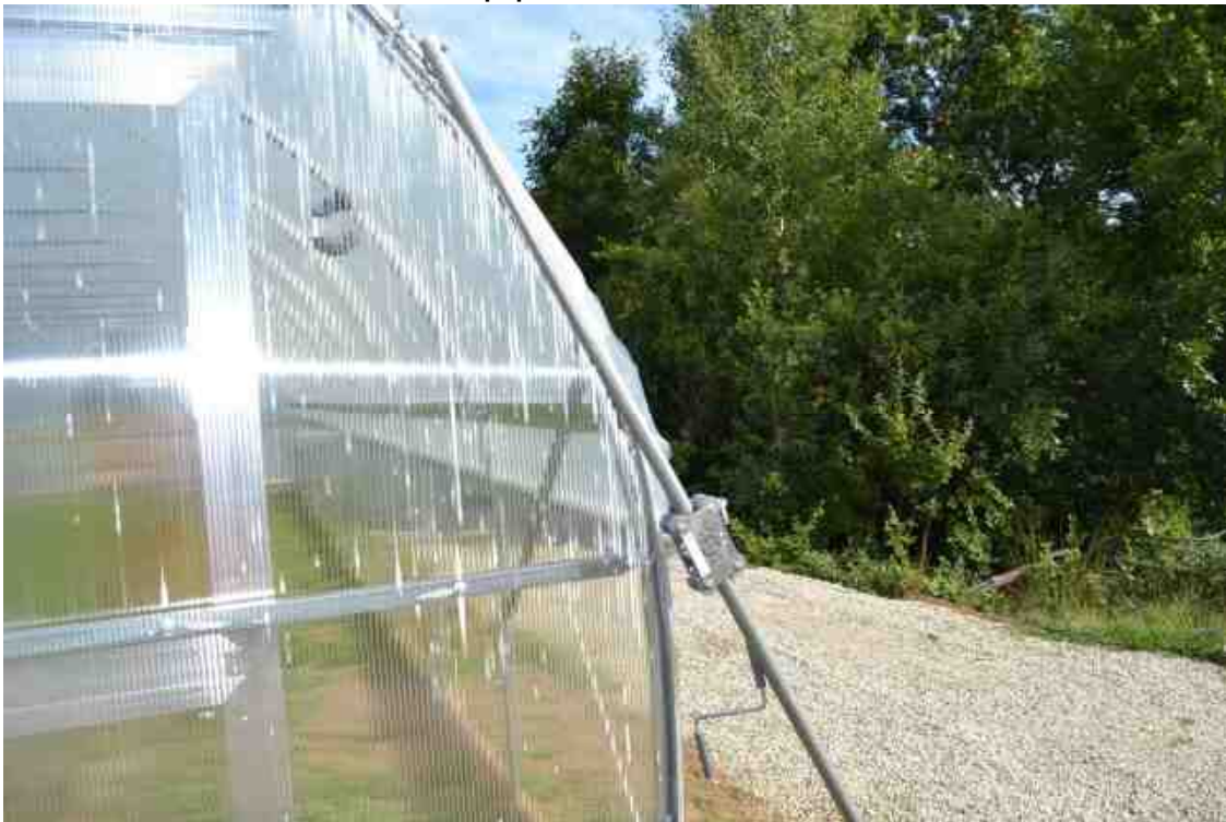
Guide pipe hardware shown
