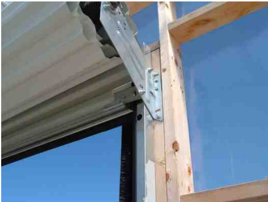
Examples of framing and installation of a roll-up door in the next series of photos
